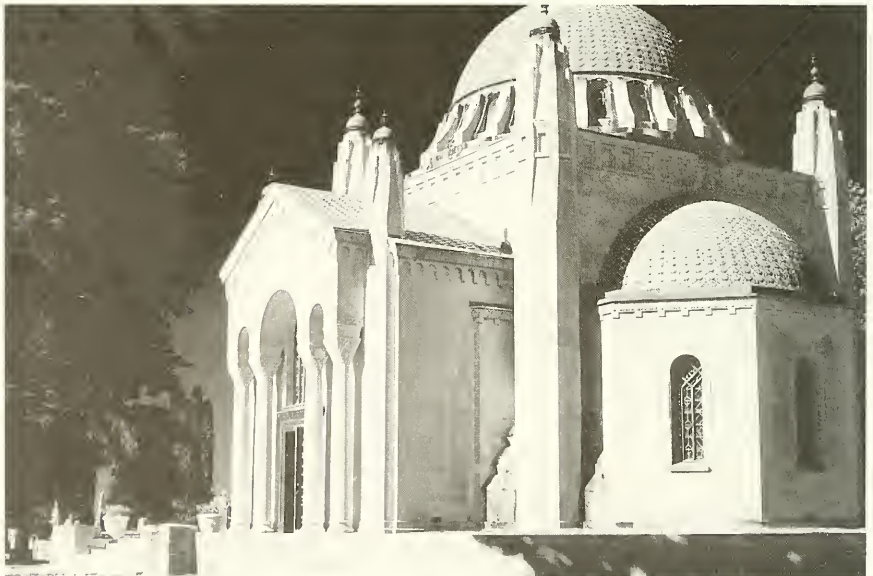
Fig. 3. Close-up, angled view of the mausoleum.
