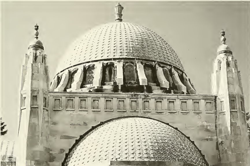
Fig. 13. Domed cupolas are roofed in patterned copper, weathered to a soft green patina.
