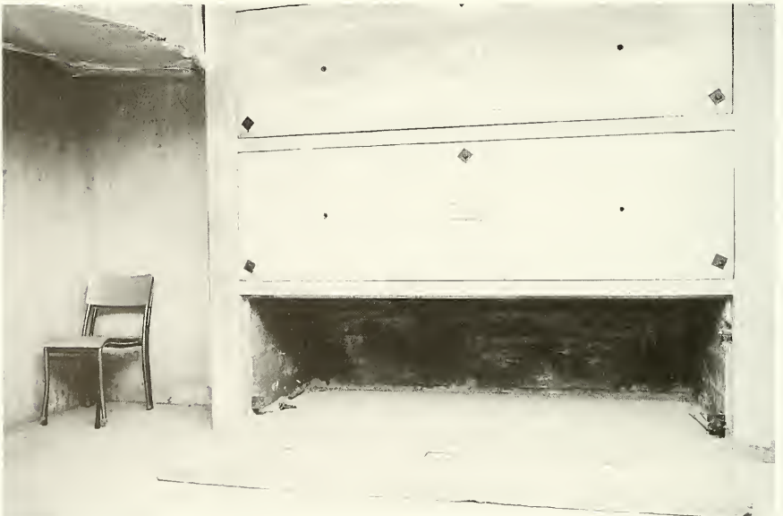
Fig. 10. Temporary storage crypts in mausoleum's sub-structure.
