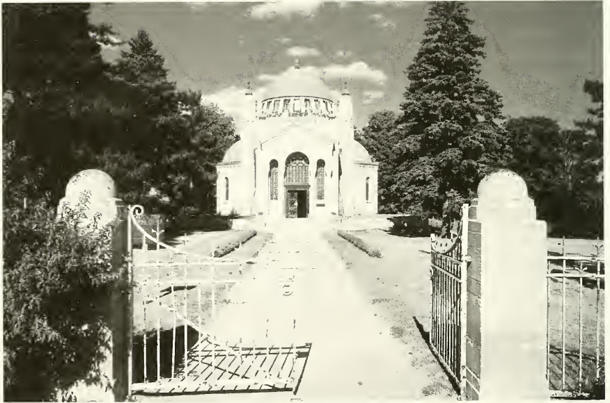
Fig. 1. Thomas Foster Memorial, Uxbridge, Ontario, Canada, as viewed from entrance gates.
