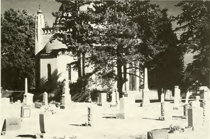
Fig. 2. Panoramic view of the Foster Memorial and adjoining Zion Cemetery.
