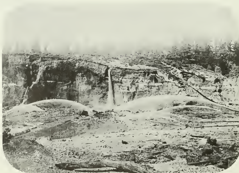
Photo 9. A Watkins photo of the Malakoff hydraulic mine as it appeared in the 1870s. This huge man-made placer-mining pit near Nevada City is today a miniature Bryce Canyon.
