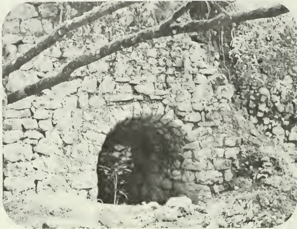
Photo 6. Olema lime kiln, built around 1850 for burning limestone from an outcrop of Calera (Franciscan) limestone. Photo by Mary Hill.
