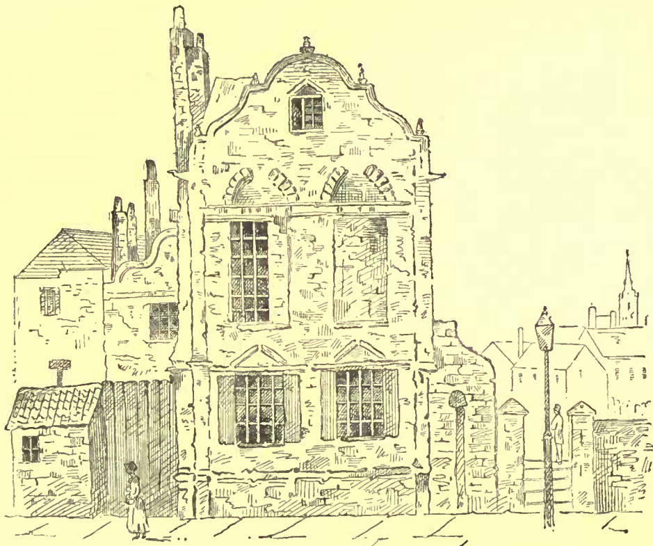
WEST END OF THE FORTH TAVERN.
