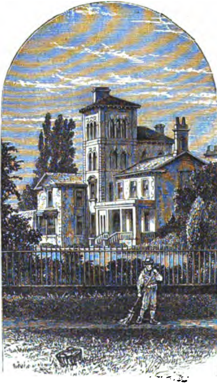
HOUSE IN CHATSWORTH PARK.
