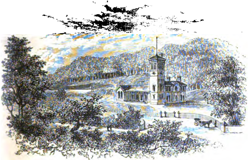
ENTRANCE TO FIRTH PARK.
